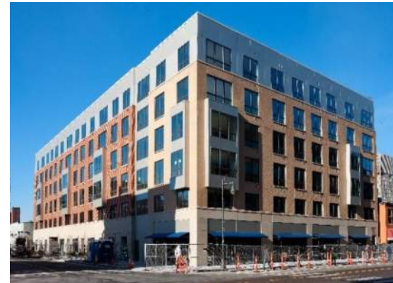
AXIOM, CAMBRIDGE, MA Construction Costs: $27,700,000 Completion Date: Oct. 2015
